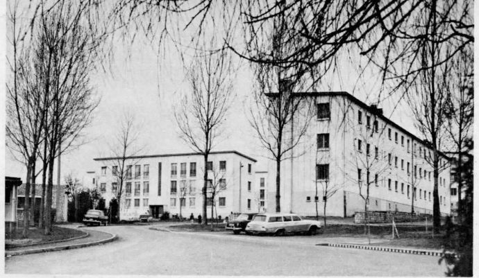
Modern government housing for the American military at St. Jean de Braye is in sharp contrast to the vintage homes and apartments of old Orleans.
