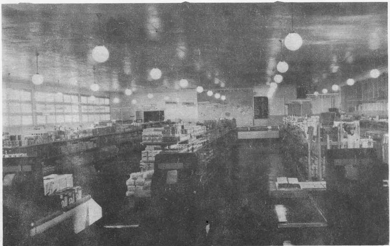
US Army Commissary Caserne Colligny
